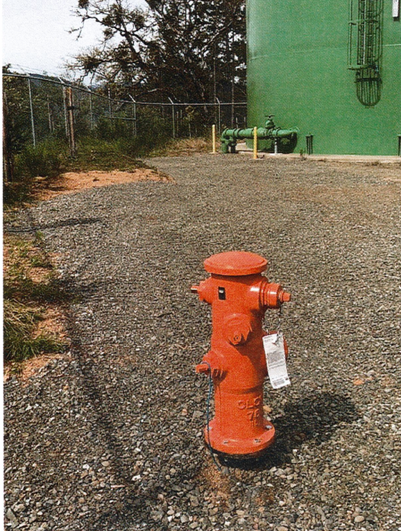
Alderpoint Rd @ Tank
