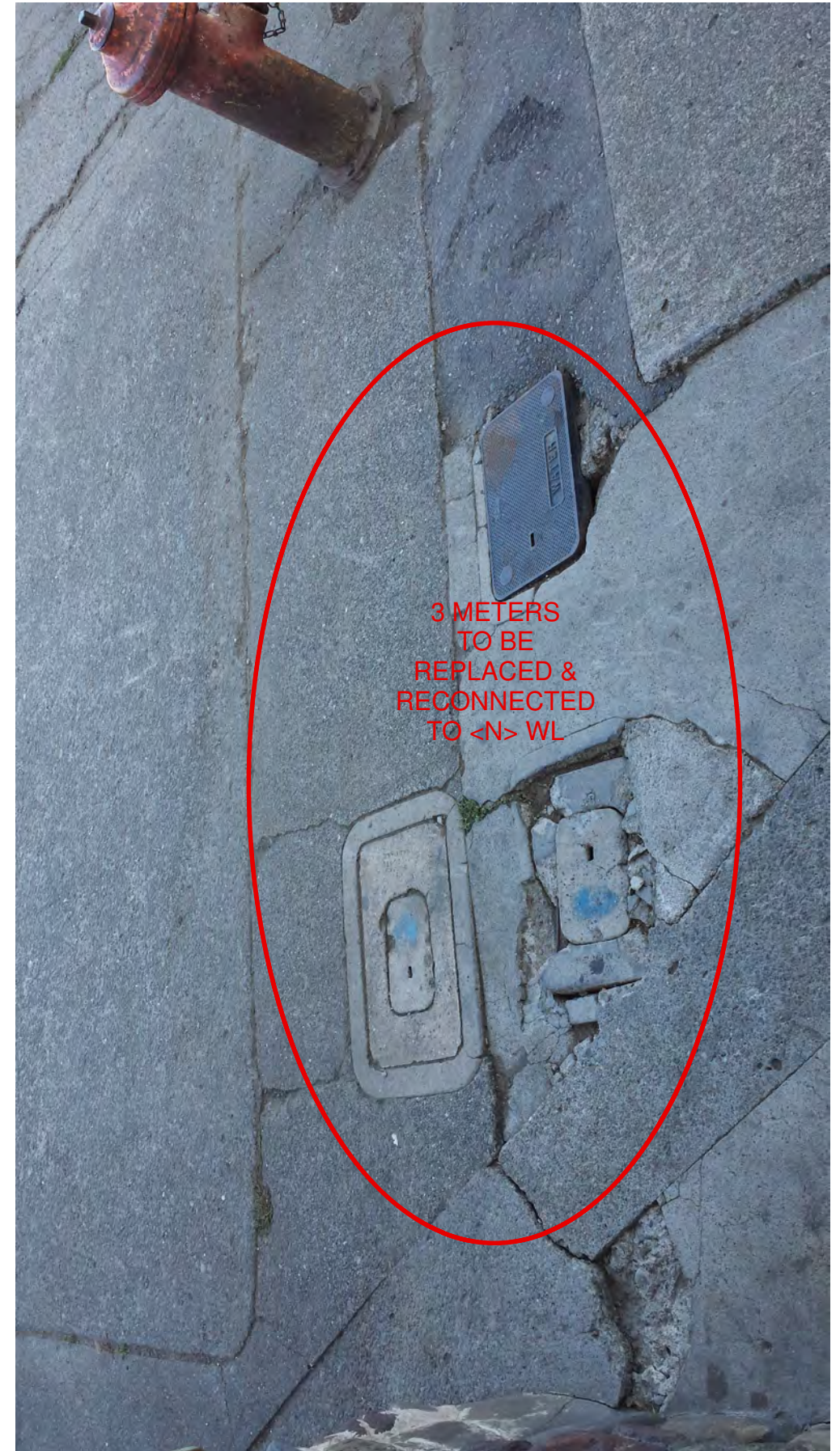
BACK OF HYDRANT
