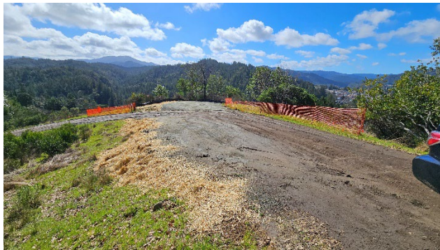
Backfilled Robertson Tank Site
