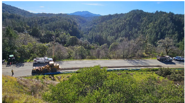
Waterline Installation in Alderpoint Road
